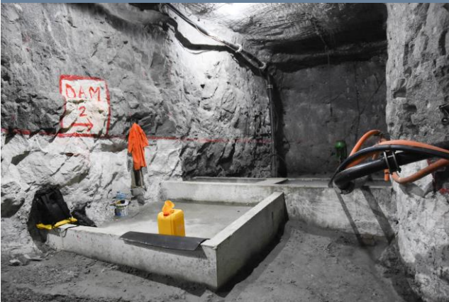
Underground Pump Station
