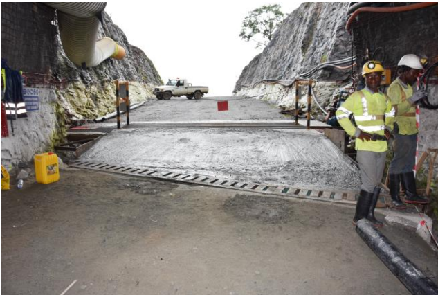
Portal entrance to the decline
