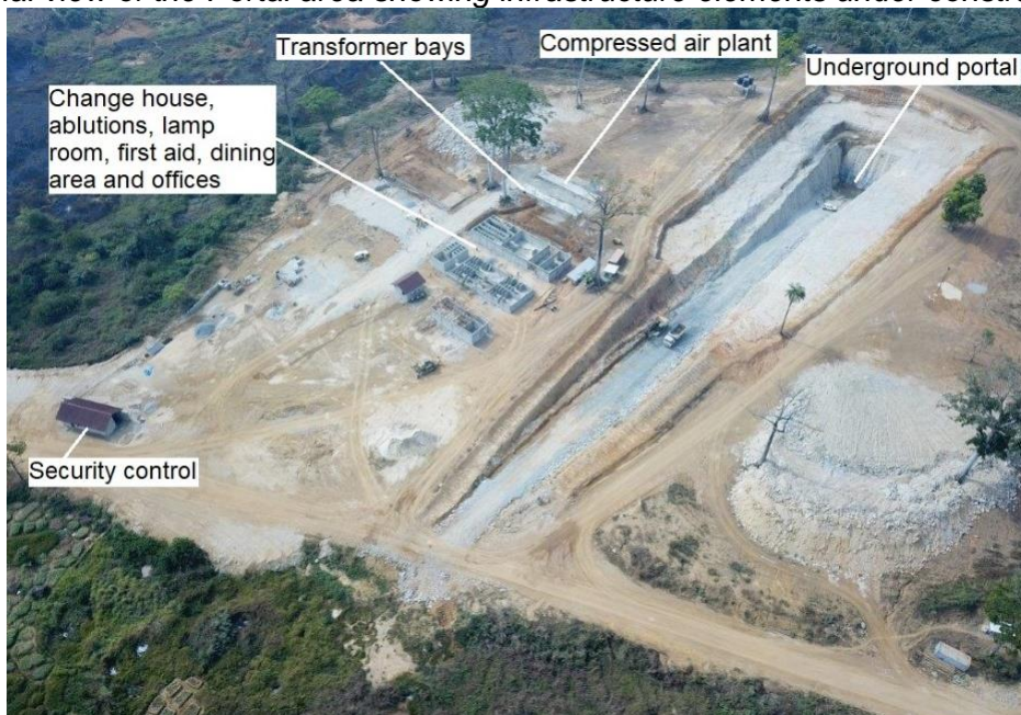
Figure 2: Aerial view of the Portal area showing infrastructure elements under construction.
