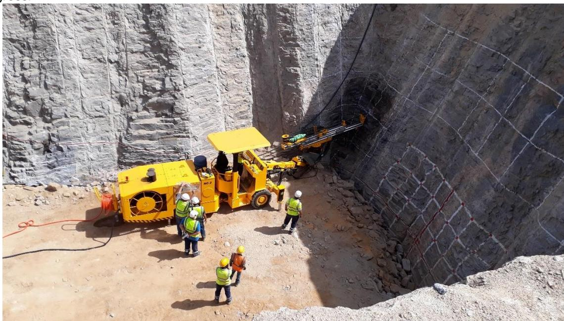
*Figure 1. Geotechnical support drilling commenced immediately after the underground drill rigs arrival and commissioning. Here we see the first geotechnical support hole being drilled in preparation for the first underground development blast.*
