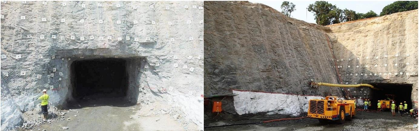
*Figure 1: Portal entrance tunnel with dimensions 6m wide by 4m high*
