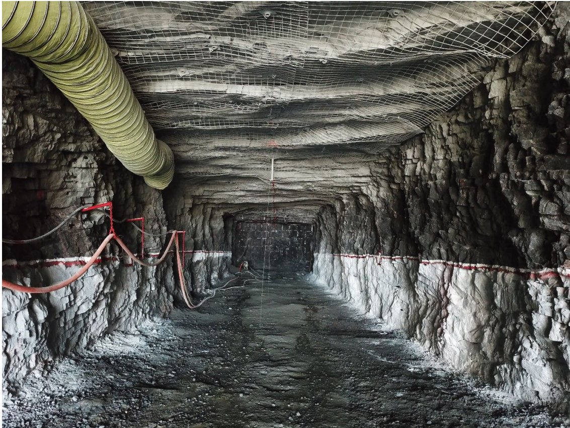
Figure 1: Underground development tunnel with dimensions 6m wide by 4m high
